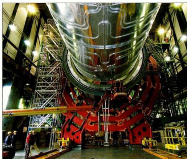
Fig. 4. Inserting the inner wall of the vacuum tank and heat shield into the 13 m-long CMS solenoid.
