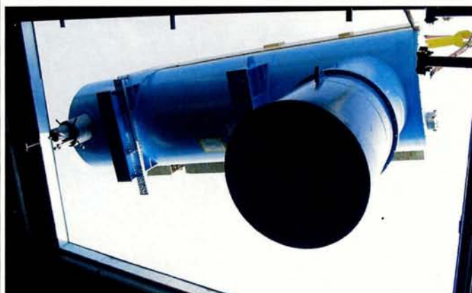
Fig. 7. A 1.8 K cold box being delivered to its underground site close to the Large Hadron Collider.
