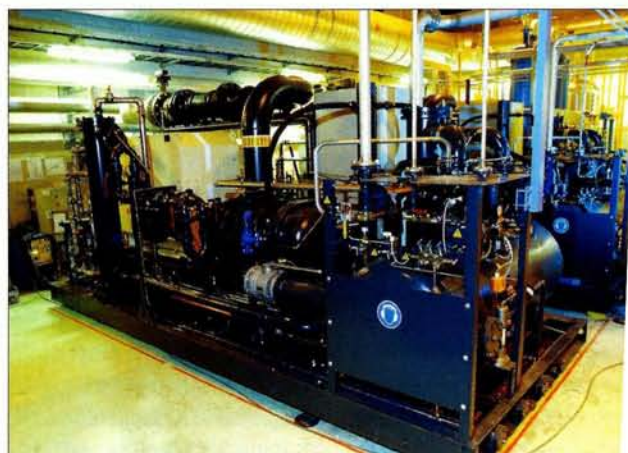
Fig. 6. The warm compressor for one of the 1.8 K refrigerator units for the Large Hadron Collider.
