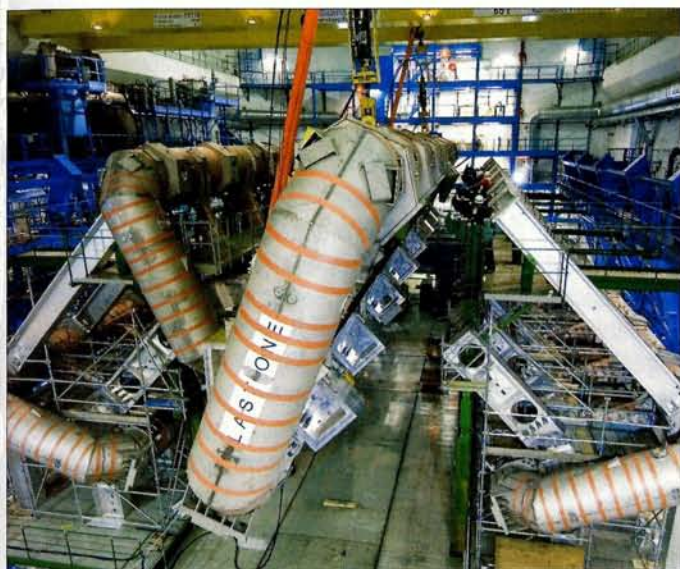
Fig. 3. Installing the eighth coil in the ATLAS barrel toroid magnet.
